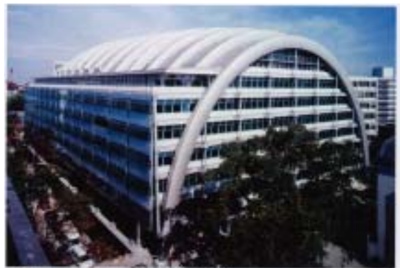
Ludwig Erhard Haus, Berlin, Germany, 1998 Stainless Steel, Seam-welded SharkSkin, AISI 316L Architect, Nicholas Grimshaw
