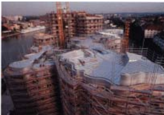
Zollhof, Dusseldorf, Germany, 1999 Stainless Steel, Seam-welded, Beight AISI 316L Architect, Frank O' Gehry
